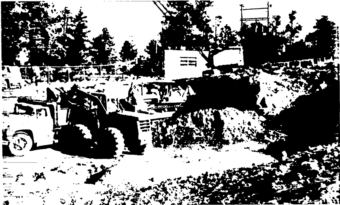
Fig. 6. Demolition and decontamination of liquid waste treatment plant.
